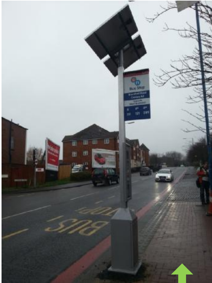
Solar powered flag poles
